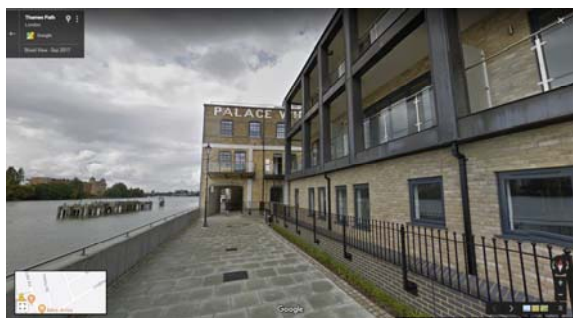
Palace Wharf, with the most recently-opened stretch of the Thames Path beneath it, is right on the current Fulham Reach-Palace Riverside boundary. The Crabtree Tavern public house is immediately to the rear.
