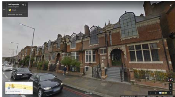
The eight artists houses on Talgarth Road currently in Fulham Reach which we propose transferring to our West Kensington ward to be in the same ward as the long terrace further behind them
