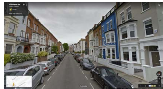
Waldemar Avenue: three storey town houses and mansion blocks: of an entirely different character to most of the area either side of the northern end of Munster Road. These Avenues lead off Fulham Road like most of the rest of Town ward does.
