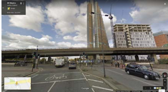
Google street view capture of Wood Lane as it passes beneath the elevated section of the Westway. This is the only point other than at the western borough boundary at Old Oak Common Lane where vehicles can cross the Westway.
