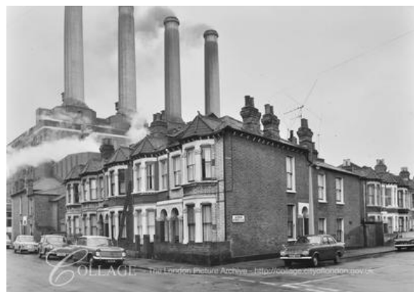
Fulham Power Station from Byam Street (credit: London Picture Archives)
