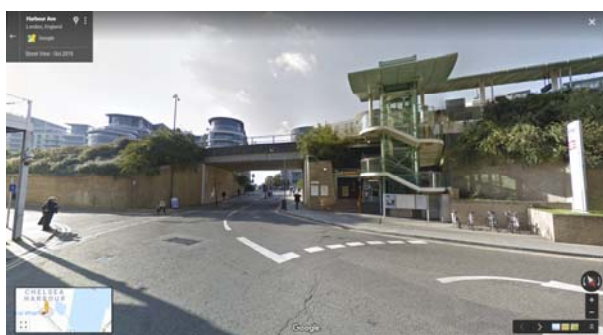
This tunnel beneath the West London Line is the only physical link between Chelsea Harbour and the rest of Fulham
