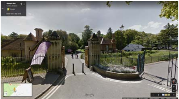
The entrance to Fulham Palace and to Bishop's Park at the end of Bishop's Avenue
